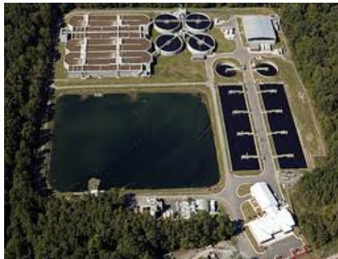
Sewage treatment plants
